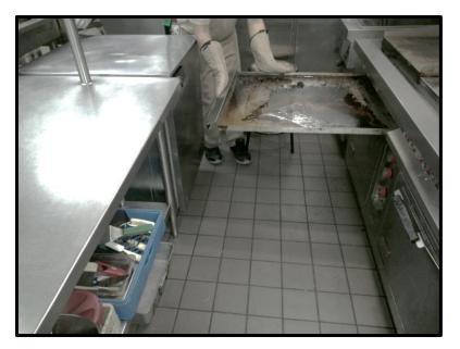
Notice that this grease trap is very dirty, and it has not been cleaned regularly. This will become a fire hazard due to the accumulation of grease and oil.
